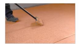
By rolling over the entire surface with a 50kg roller when installation is complete
